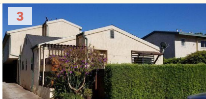
3 2458 Barry Avenue West Los Angeles $1,700,000
